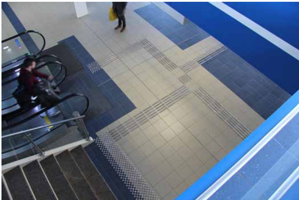
Trnava Train Station, Slovakia. Stainless steel with diamond/pyramidal surface.
