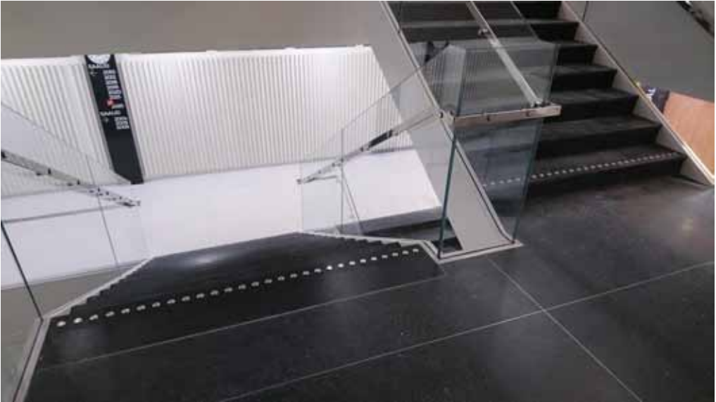
County Court Harju, Tallinn, Estonia. The stairs are marked with self-adhesive studs.
