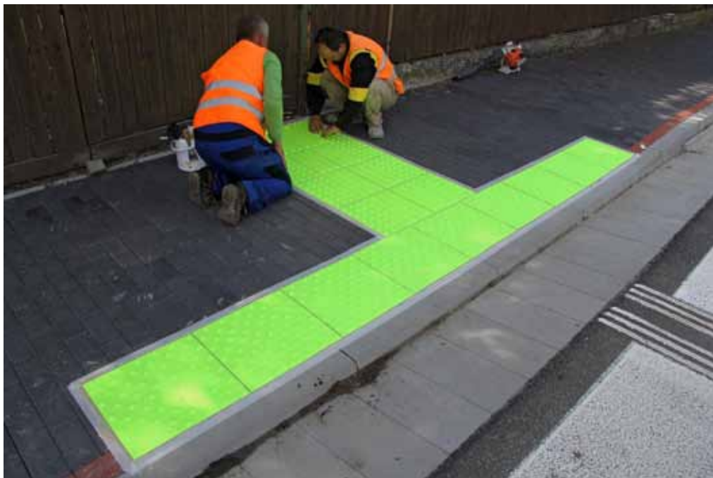
Budimír, Košice-okolie, Slovakia. Installation of polyurethane plates in reflective green.
