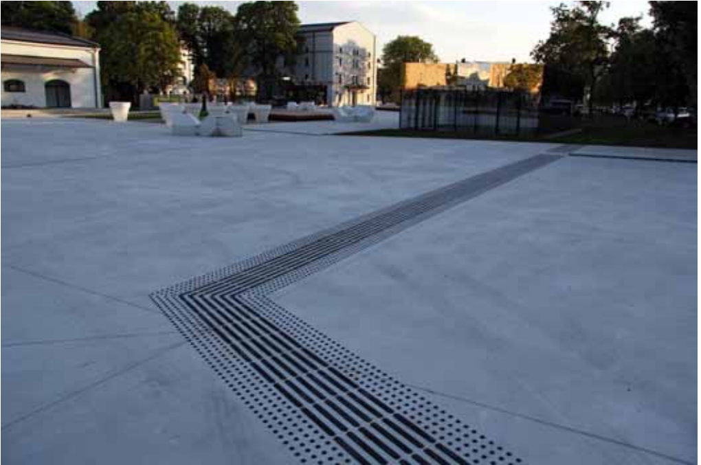
Kulturpark Košice, Slovakia. Polyurethane floor indicators can likewise be drilled in.
