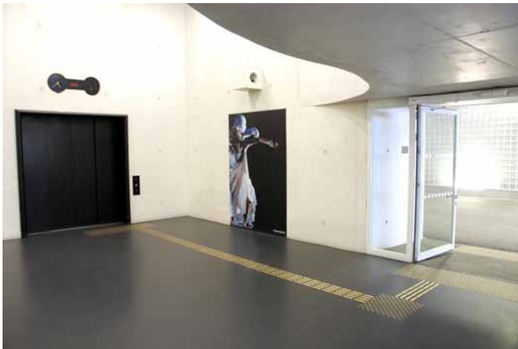
State Theater Darmstadt, Germany. Brass guiding system, drilling installation.
