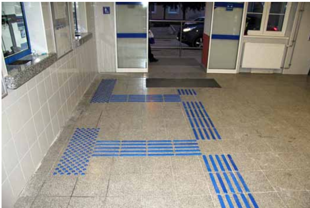
Trenčianska Teplá Train Station, Slovakia. Self-adhesive strips and studs from polyurethane.
