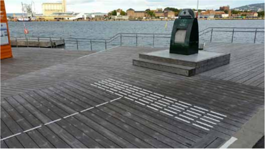
Sørenga brygge, Oslo, Norway. Steel strips with colour polyurethane inserts.
